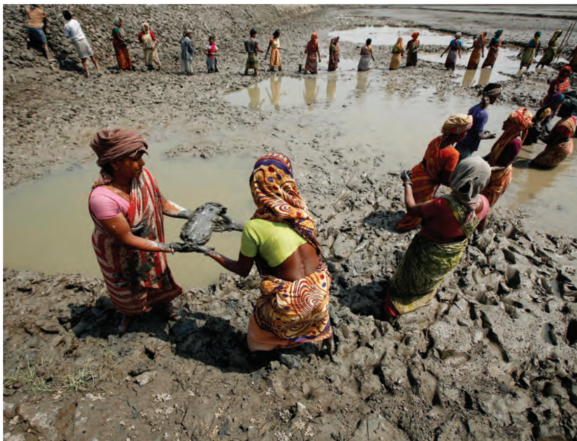
Women work to rebuild an embankment in one of the regions hit by Cyclone Aila in Dacope, Khulna, Bangladesh.
